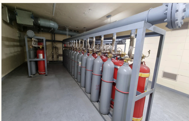
gaseous fire-extinguishing agent bottles
